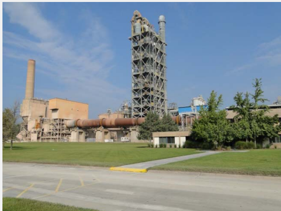
Overview of new line
