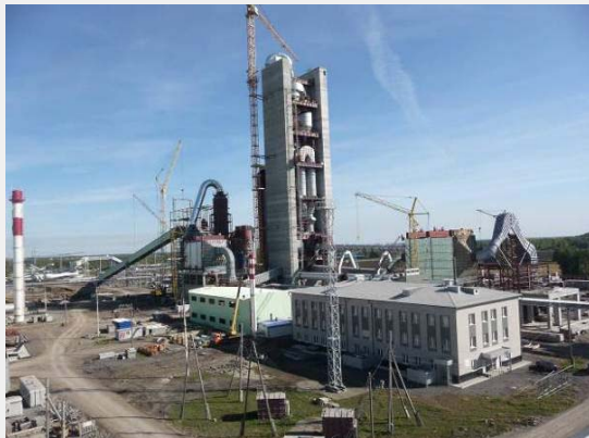
Overview of new line
