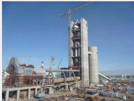
Tower and kiln basement
